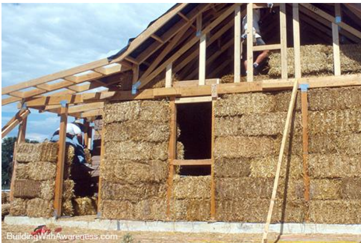
Figure 8. Straw Bales Building Material 9
