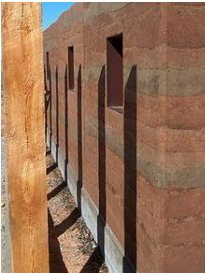
Figure 7. Rammed Earth Wall 7
